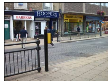
Raised and signalised crossing in Biggleswade
